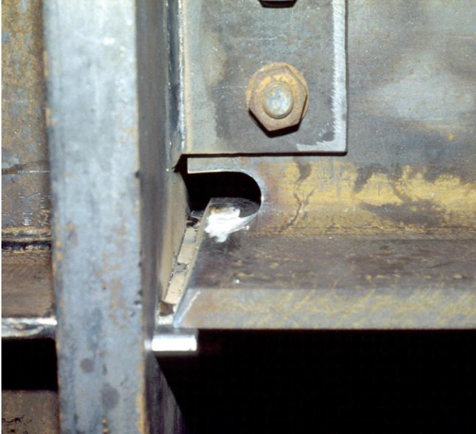
Root, Weld Access hole, Bevel, Backing Bar
